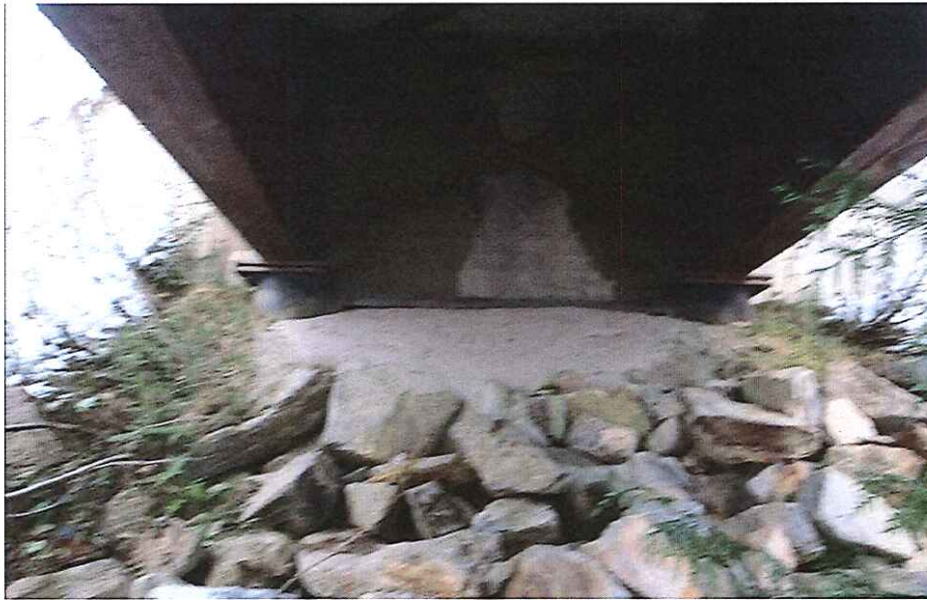
CK2356 Right abutment
