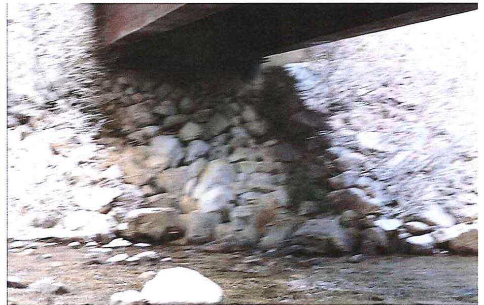
CK2356 Left abutment
